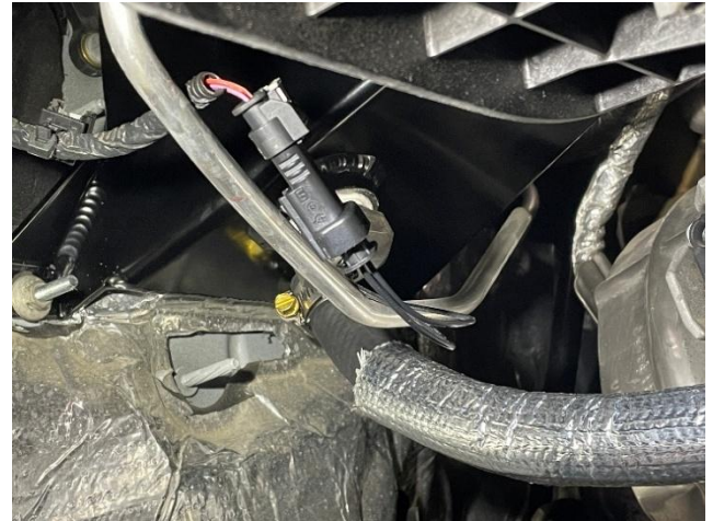
Figure 32: New coolant level switch plugged in.
