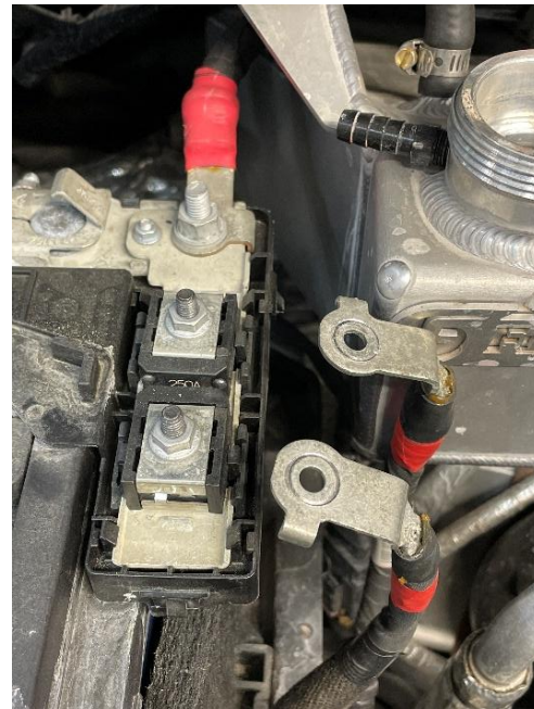
Figure 11: Removal of each auxiliary cable from the positive terminal.
