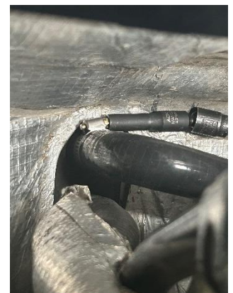
Figure 11B: Installation of supplied hose clamp at firewall.
