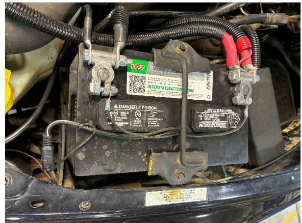
Figure 8: Negative battery terminal reinstalled.
