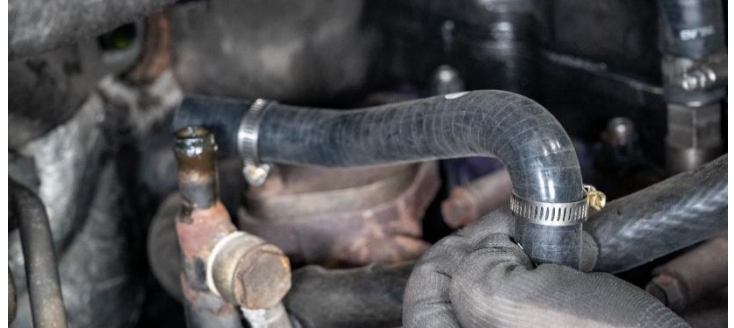
Figure 6: Installation of new Fleece heater core hose.
