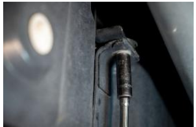
Figure 18: Reinstallation of fuel tank straps.
