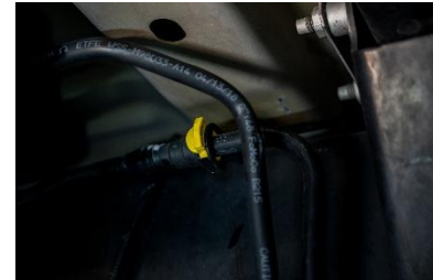
Figure 21: Reinstallation of fuel feed line.
