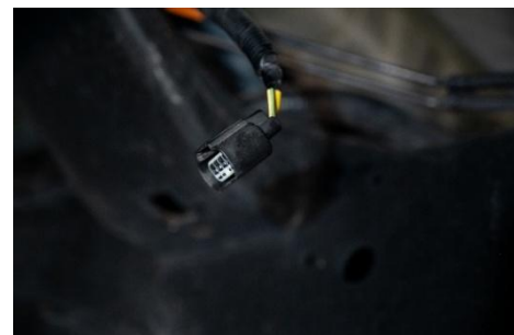
Figure 8: Stock lift pump electrical harness disconnected.
